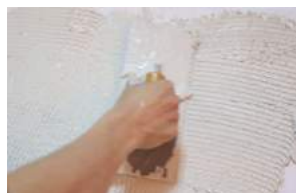
4. Apply the adhesives to the substrates
